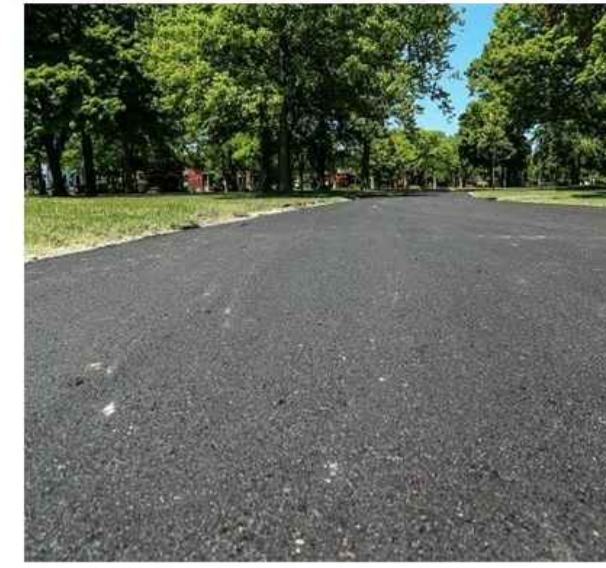
02 Asphalt surface to paths
